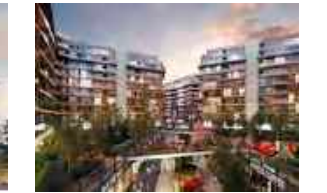
Lens İstanbul Property type: Residential Developer: Lens Construction Residences: 982
