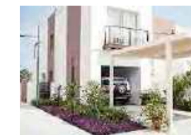
Al Mouj, Wave Muscat Property type: Residential Date opened: 2018/2019 Developer: Al Mouj Muscat Residences: 140
