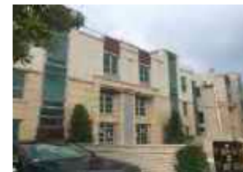
Kadoorie Villas Property type: Residential Developer: Wing Shing
