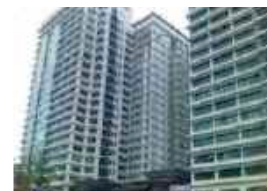
North Point Condominium Property type: Residential Developer: IGB corporation Residences: 300
