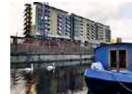
Suttons Wharf North Property type: Residential Developer: Hollybrook Number of residences: 450
