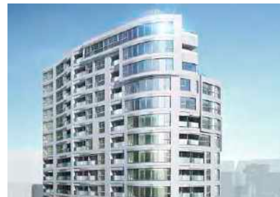
The Conoe Daikanyama Property type: Residential Developer: APA Home Residences: 109
