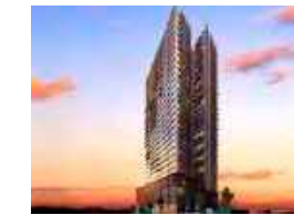
Air Apartments Property type: Residential
