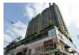
Commune Modern Property type: Residential Developer: Sino Land Company Ltd. Number of residences: 296
