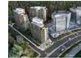
Vadi Kuru Property type: Residential Developer: Invest Construction Residences: 288
