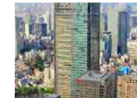
Tokyo Mid Town Property type: Residential Developer: Mitsui Fudosan Residences: 166
