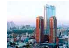
Roppongi Hills Residence Property type: Residential Developer: Mori Living, Todakensetsu, Shimizu Seibu Kyoudo Jigyouta Residences: 793
